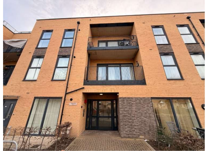
DA8 1AR, Elliston House West Street
