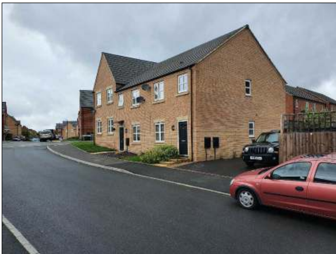
CV3 1QG - David Spencer Drive
